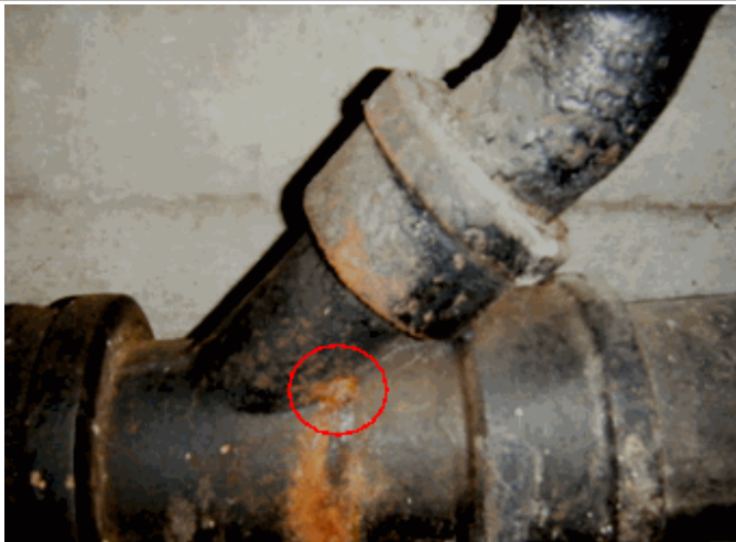
Corrosion on drain pipe from pin hole leak; replace drain pipe
