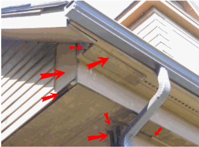
Exterior: Missing molding outside
