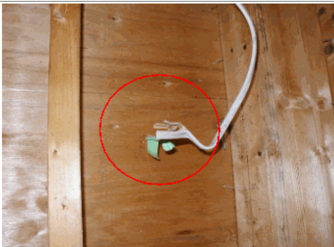
Elect.: Terminate free end wires in boxes, this one in garage one under window in bedr
