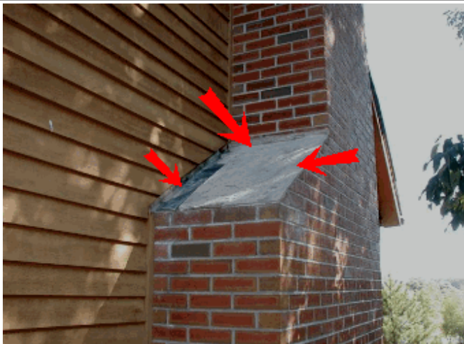
Exterior: Flag stone missing from chimney
