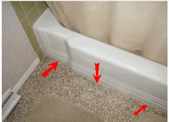
Seal between tub and floor to avoid floor damage.
