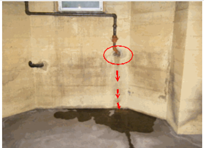
Water leaking into basement; seal around gas pipe & correct yard drainage to reduce
