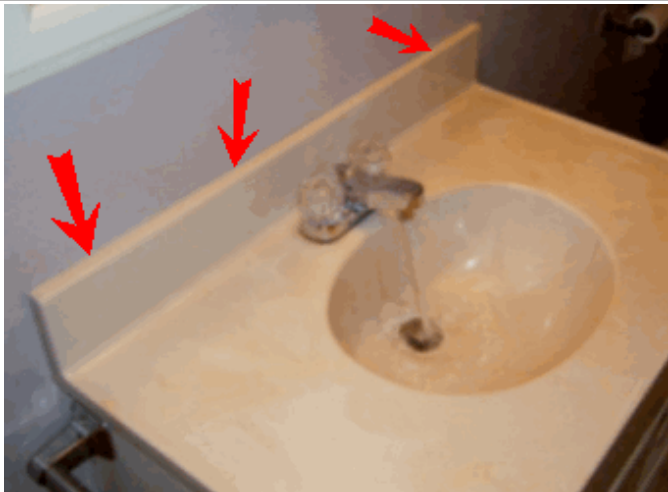
Seal between sink countertop and wall
