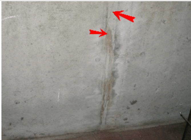
Crack in foundation wall is NOT a structural concern, some water weeps in
